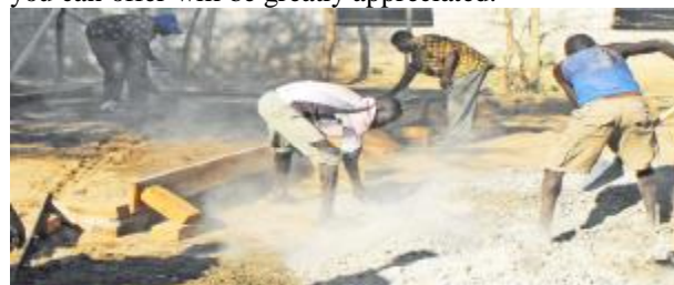
"Pouring" the slab for the new kitchen and library
